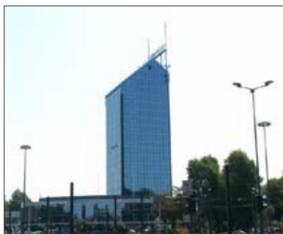
Błekitek, now re-named K1, is the tallest office building in Krakow. The K1 building will be extensively refurbished and modernised.
