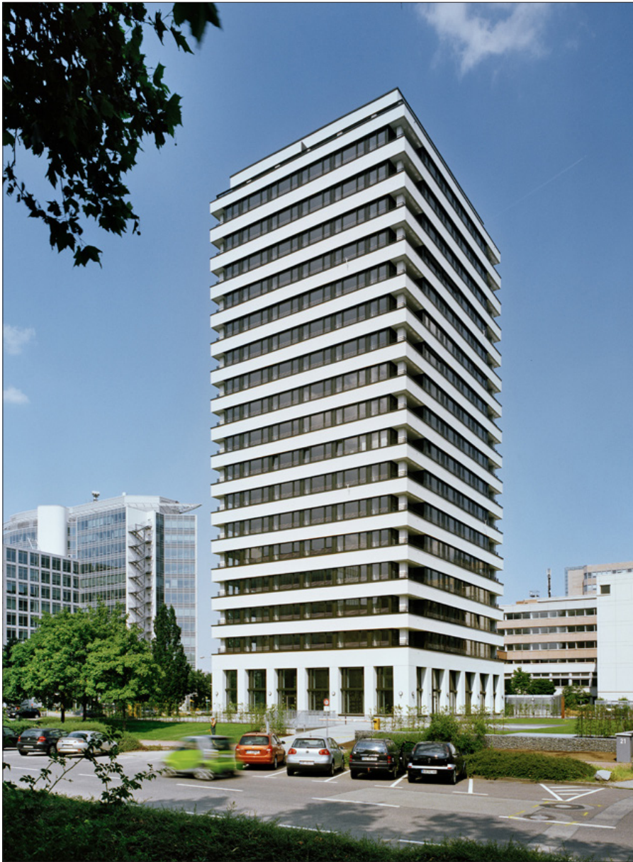
The Niederrad office district in Frankfurt am Main is now a mixed-use neighbourhood.
