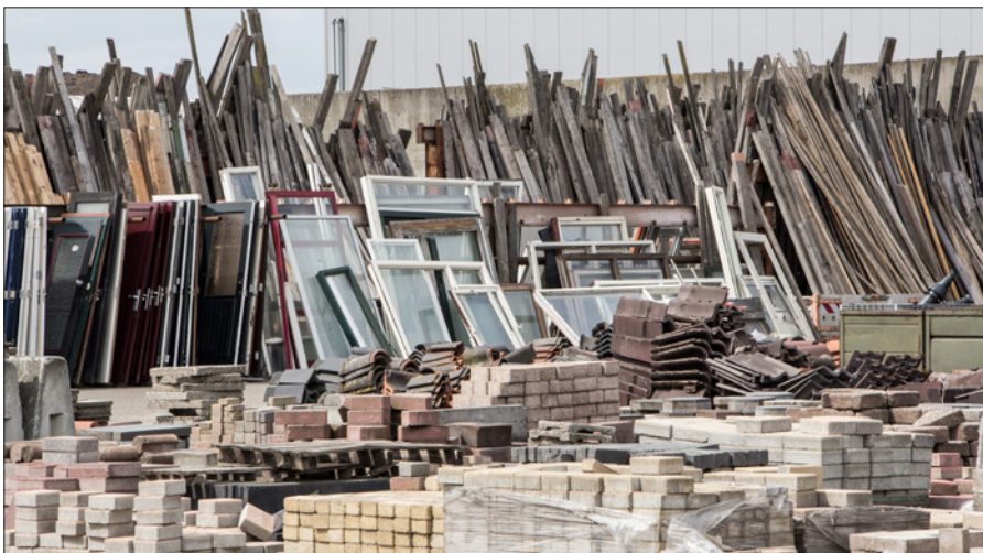
Recycling demolition materials helps to save energy and resources.
