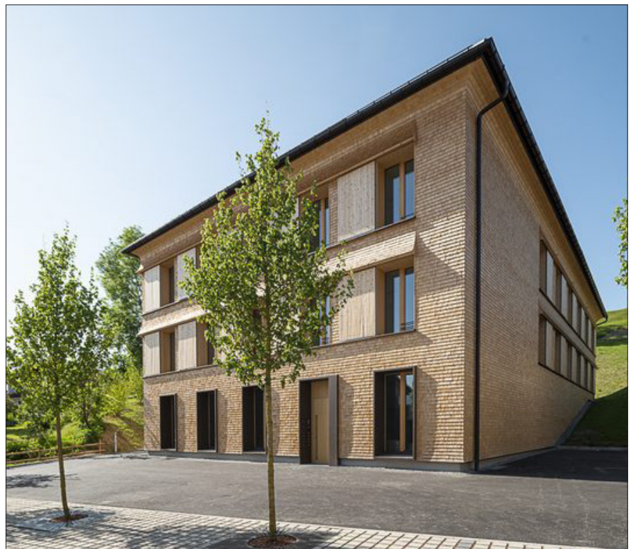
Therapy rooms, office space and four residential units – heating not necessary
