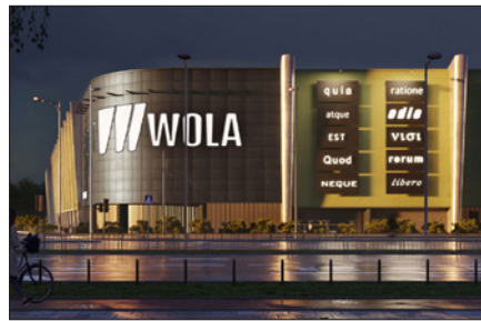
After an interruption of six years Fort Wola shopping centre has been reopened.
