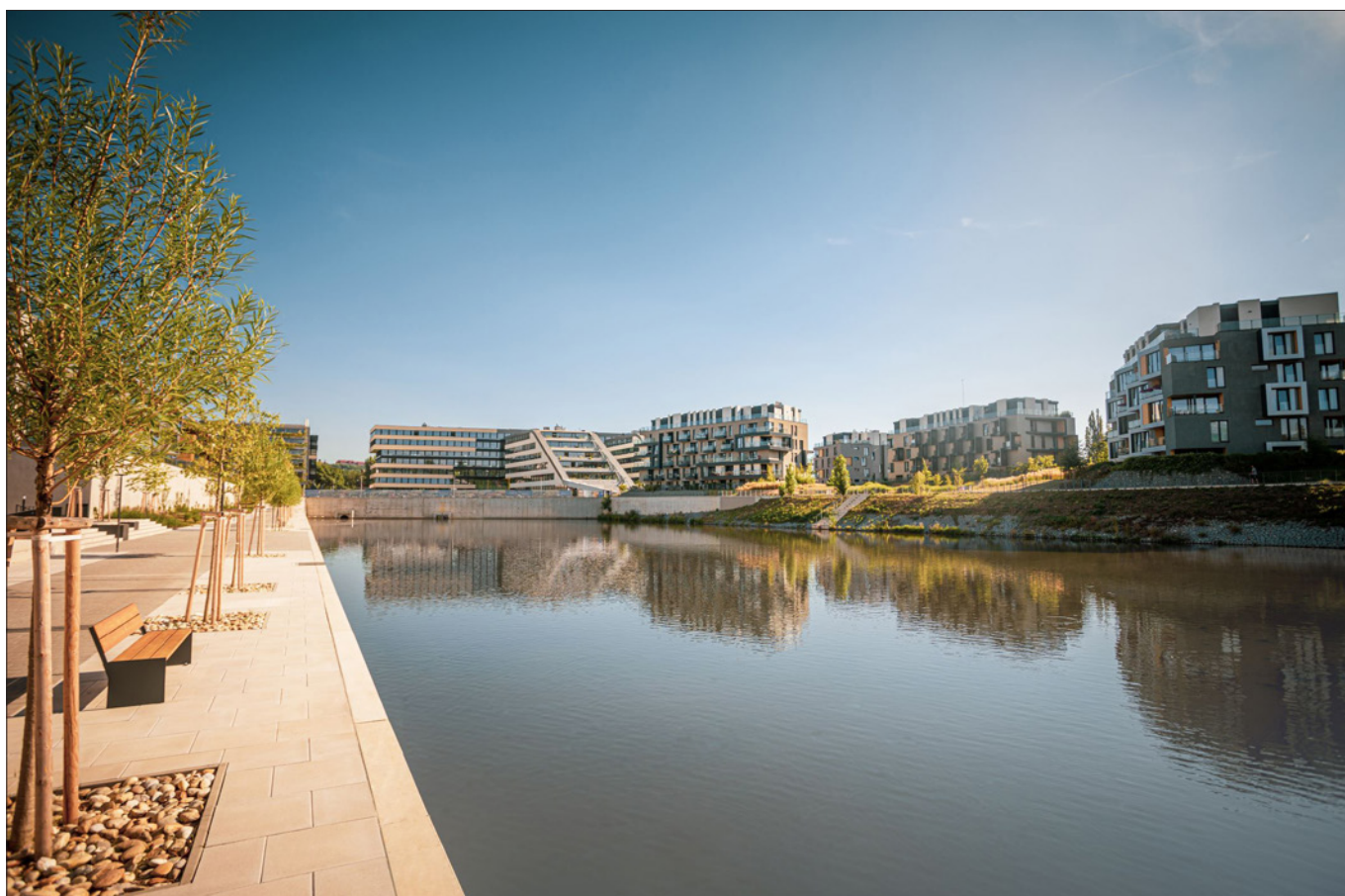
One of the major urban development projects in Prague: Dock, the conversion of a port area on a distributary of the Vltava.
